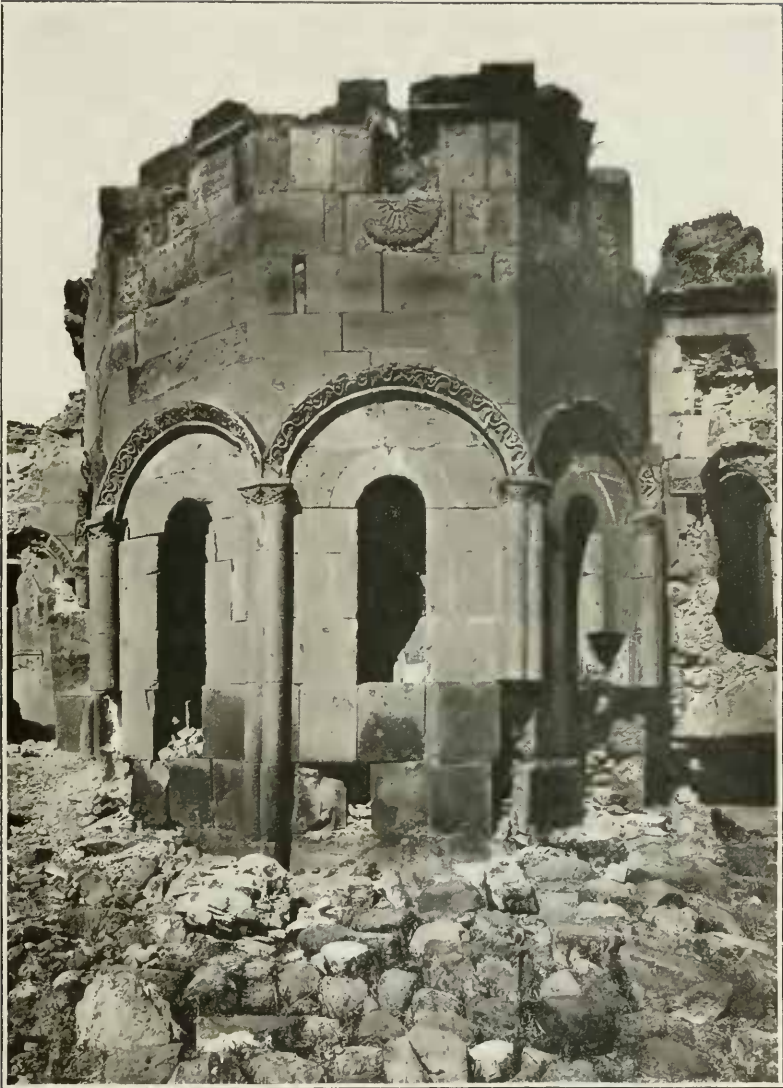
FIG. 62. TALIN: MOULDINGS ON SOUTH SIDE OF RUINOUS CHURCH.
