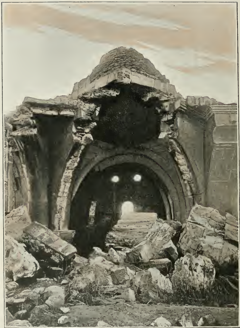
FIG. 91. ANI: PORTAL OF THE CHURCH OF THE APOSTLES FROM THE WEST.
